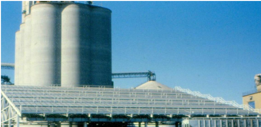
Figure 8. A large-scale forced convection solar dryer
