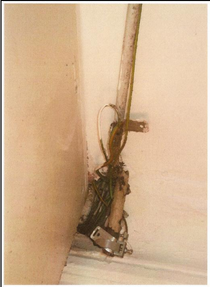
Figure 8.4.11 – Earth clamp connection
