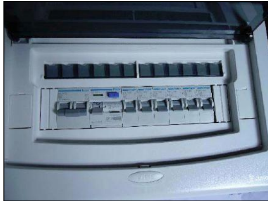
Figure 5.8.3 – Diagram of a distribution board in a domestic dwelling
