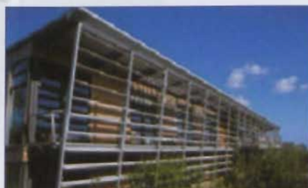
Figure 5 — Example of external louvre solutions
