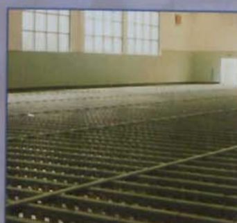
Sprung flooring systems for sports hall. Polysport®
