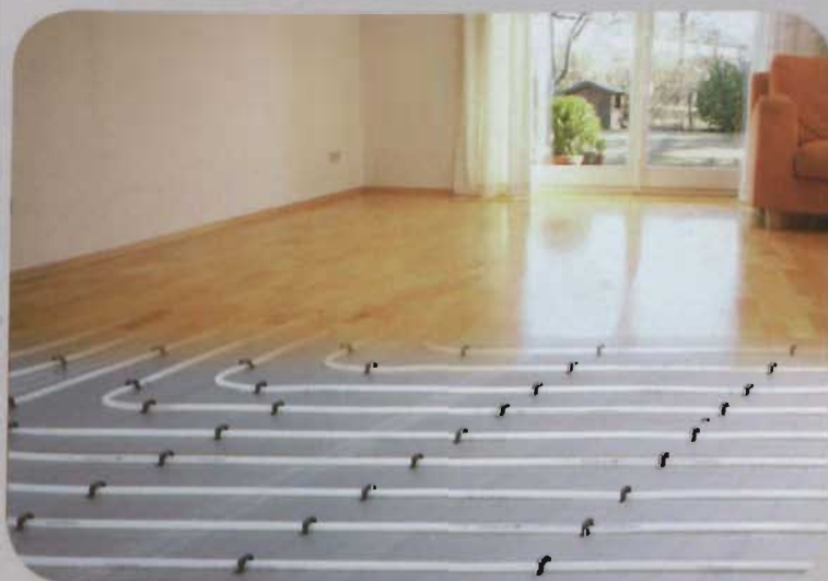
Multilayer pipe system with staples
