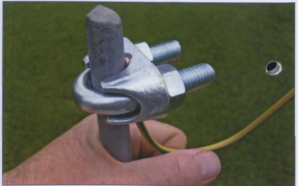
Figure 1 — A Typical Rod Earth Electrode
