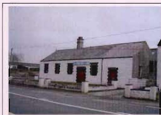
Fig 21: Drumcliff Creamery Building Milltown
