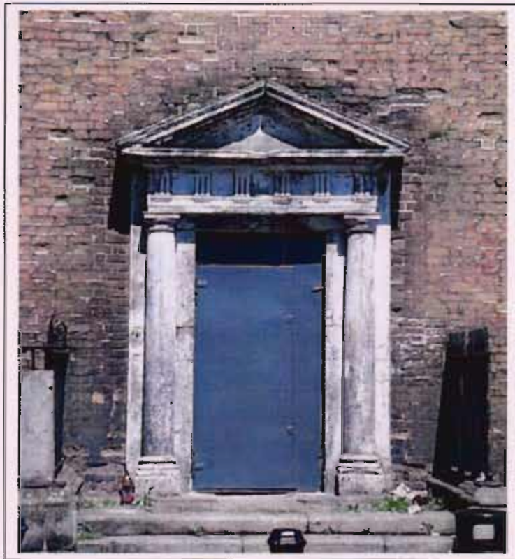
Fig 129: Portland stone doorcase to No 3
