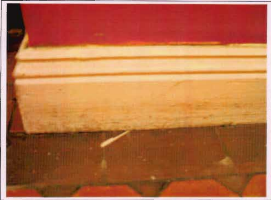
Fig 76: Detail of timber moulded skirting to entrance hall
