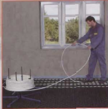
Pipe Laying with Adjustable Pipe Decoiler
