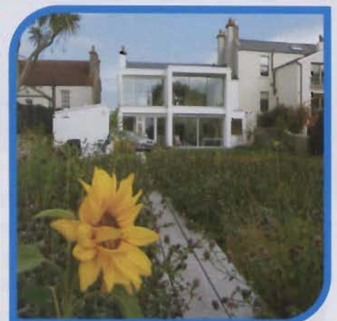
Harnessing Nature's Heat - House Design by Fitzpatrick & Mays Architects
