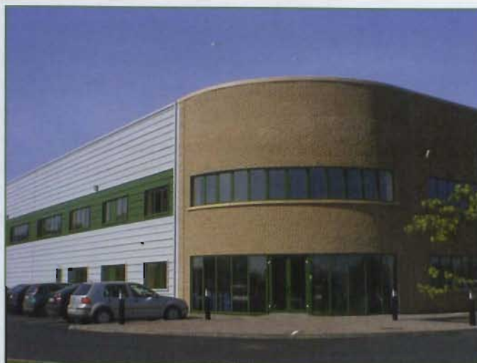
Cylon's headquarters in Dublin is fitted out using the company's own state-of-the-art building management control systems.
