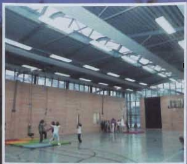
zehnder radiant ceiling panels
