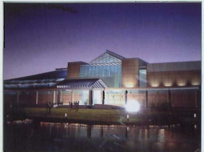
In addition to prestigious installations in Ireland and throughout Europe, Cylon building management control systems feature in high profile projects throughout the world. A typical example is the Fangfeiuyan, Diaoyutai, State Guest House pictured above. This is where China hosted the North Korean nuclear talks.
