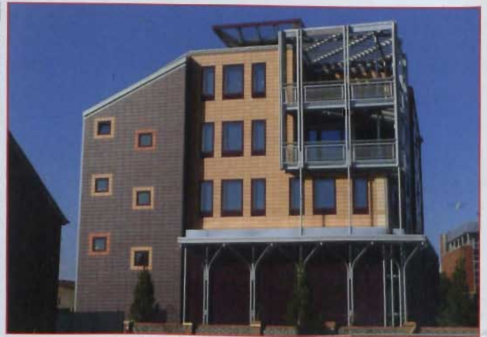
The Navan Credit Union Offices, Navan, Co Meath where Crystal Air have just completed the installation of a new gas engine heat pump air conditioning system.
