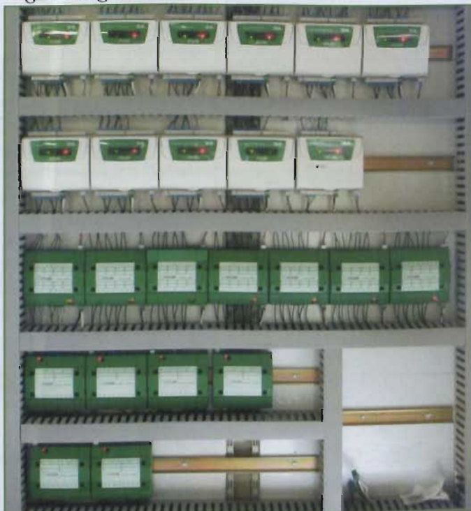
The smaller form factor of UnitronUC32 products reduces the size of MCC panel required
