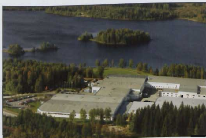
This demonstrates the scale of Systemair's headquarters in Sweden
