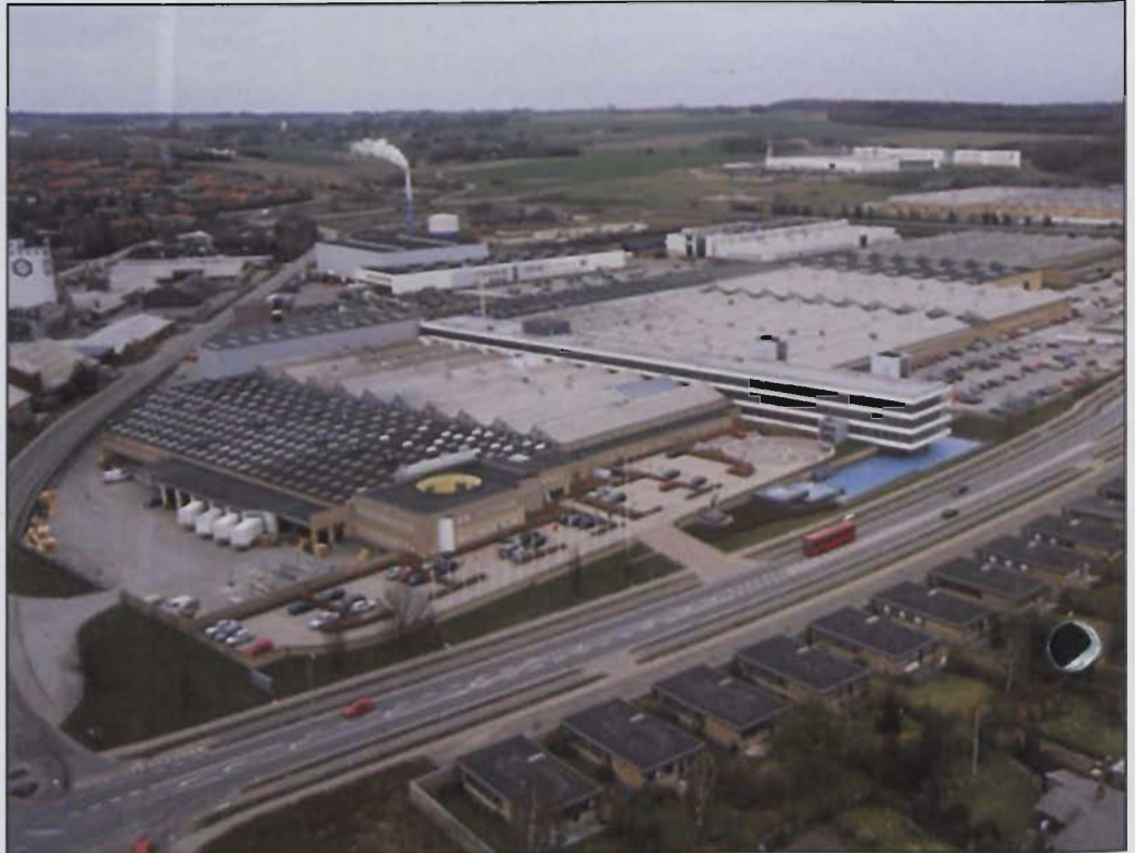
The massive Grundfos manufacturing facility in Hungary
