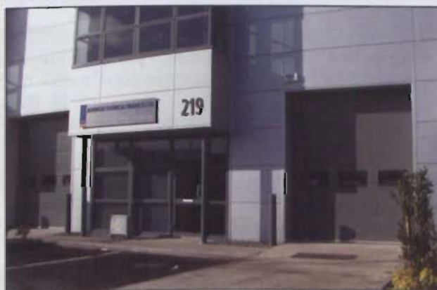
ATP's purpose-designed premises in Ballycoolin, Dublin
