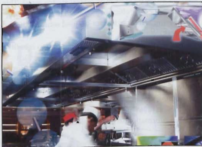
The Halton Capture Ray system exposes cooking effluent to UV light, which breaks down grease molecules into smaller harmless molecules
