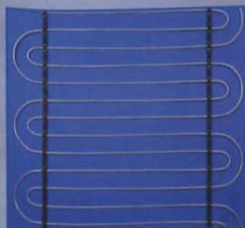
Wall heating using pre-assembly units.
