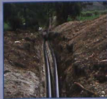
District Heating — pre-insulated pipes. Calpex®
