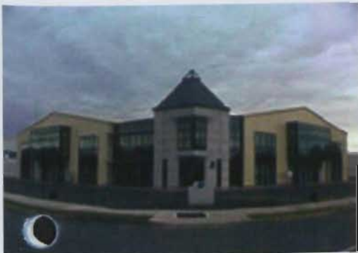
Unico System Ireland Offices, Mullingar, Co Westmeath
