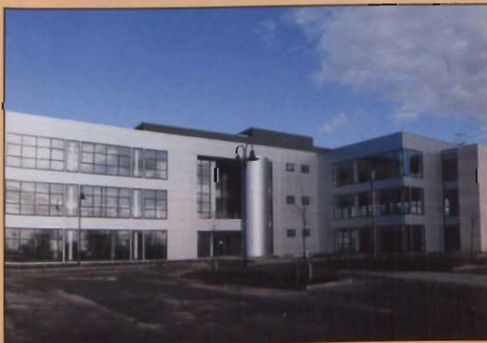
Millenium Park — In one of the first installations of its type in the country, a new type Mitsubishi Electric VRF system was installed by Tony Harmon Services Ltd
