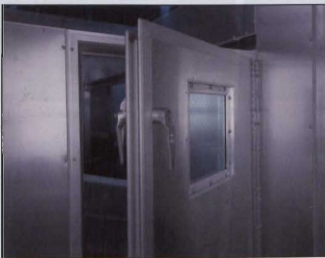
Integral casing mullions provide component mounting within the unit without penetrating the casing. Air quality, and air and vapour leakage integrity, are not compromised.
