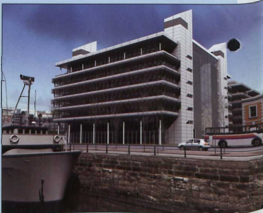
Schematic of PriceWaterhouseCooper's new 300,000 sq ft headquarters for which Treasury Holdings has just received planning permission
