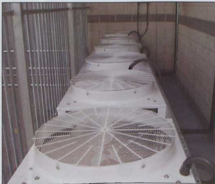
The Sanyo W Eco multi outdoor units serving the UR ducted indoor units at Elverys new superstore in Dublin.
