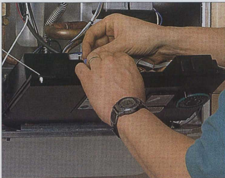
The drop-down control box provides easy access to all components, facilitating service work.
