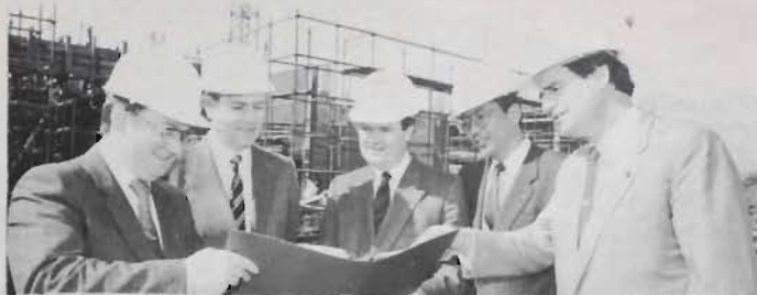
• New Dublin Gas has won the contract to supply natural gas to Yamanouchi Ireland Co Ltd, in Mulhuddart, County Dublin. Pictured on site at Yamanouchi were (from left to right): Paul O'Shaughnessy, General Sales Manager, New Dublin Gas; Bernard Somers, Receiver and Manager, New Dublin Gas; Colm Regan, Divisional Manager, Industrial Development Authority; Isao Kishi, Manager Plant Construction, Yamanouchi; Joe Harford, General Manager, Yamanouchi Ireland.
