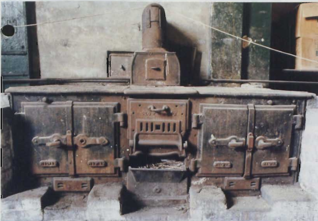
● Pictured above is an original Glow-worm double oven cooking range which dates from 1932. When discovered in an unused kitchen area of a large Grade 1 listed building in Norfolk, England, it was found to be in perfect working order.
