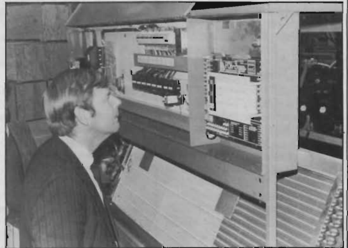
● Above: Brian Carlile, ESB, Cork with Peter Kelly, also from the ESB Cork office. Above right: John Sweeting, Cork Gas with Larry Sheerin, Limerick Gas and Peter Michaels, Cork Gas. Right: Barry Leach inspecting the air-conditioning unit at Liebert International.
