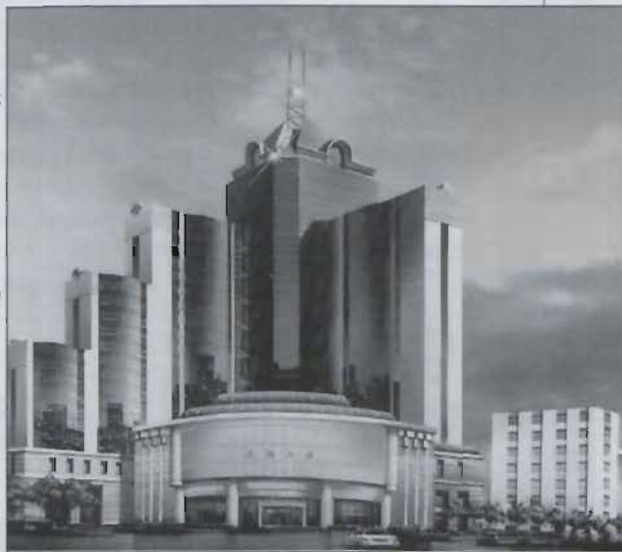
Cheng Ming Mansion, Beijing, Republic of China which will incorporate Cylon Unitron building management systems
