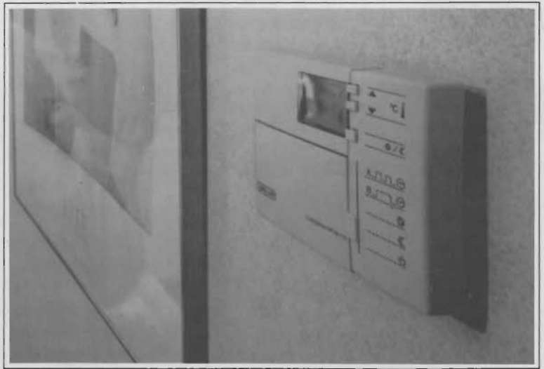
The new Landis & Gyr Chronogyr REV 10 programmable room thermostat for central heating control. Details from ASEA Brown Boveri.
