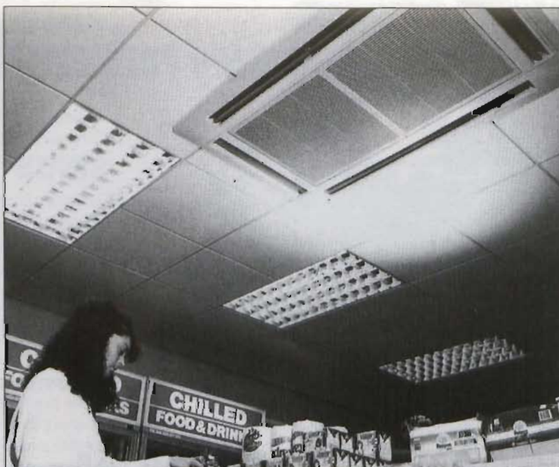
Typical retail application of a Mitsubishi Electric split air conditioning system
