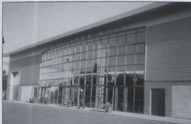
Left: The Shelbourne Hall, RDS, where Mark Éire was responsible for the entire heating and ventilation system.
