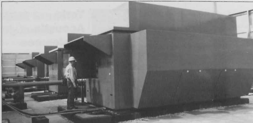
An example of the Phase 5 Acoustic Kit developed by York ACR in conjunction with Conabears Acoustics.
