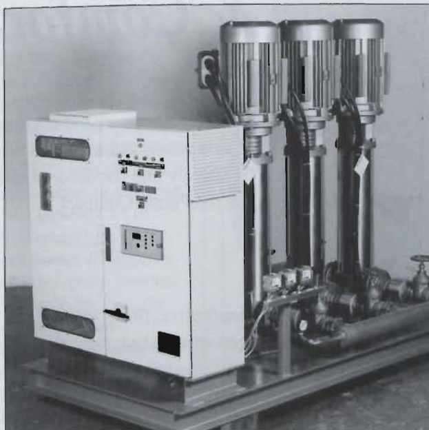
Holpak 3-pump variable speed packaged pumpset, as designed and manufactured by Holfeld Pumps. This particular unit is installed in a high-profile international hotel in Dublin.
