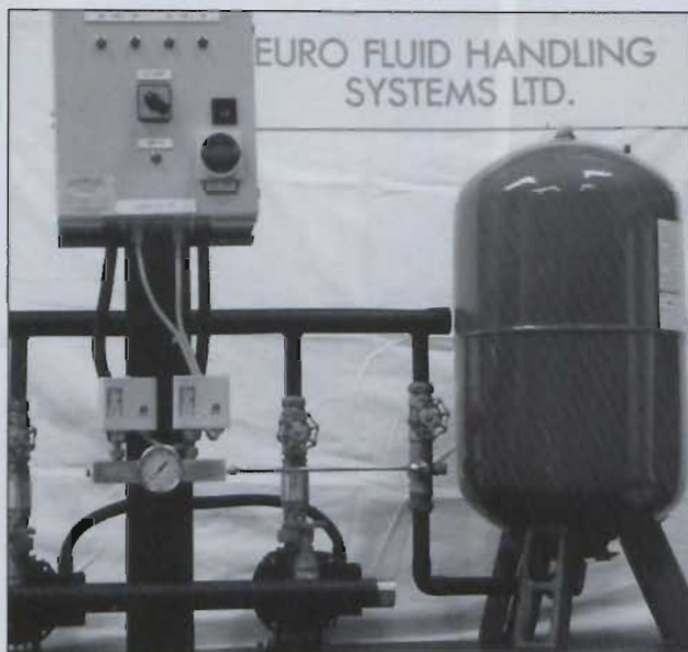
Eurofluid mains water and cold water duty assist booster set
