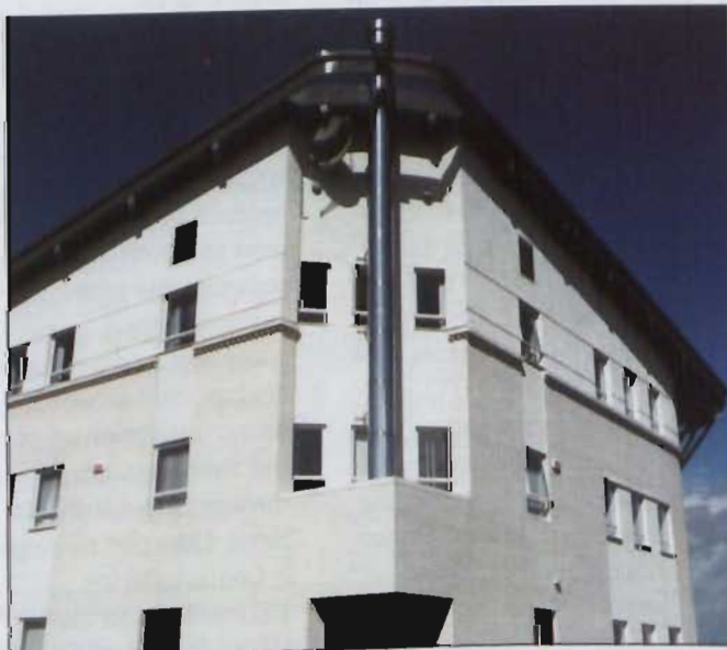
IC(A)L T.30 Chimney at Fiat (Irl) Ltd
