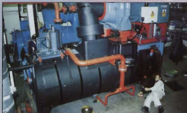
Installing new shell insulation
