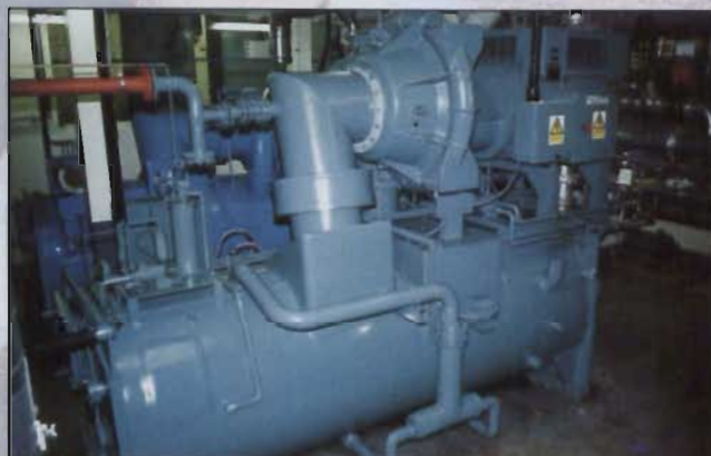
The completed retrofitted unit with new York Driveline
