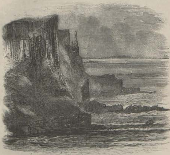
CHIMNEY TOPS, GIANT'S CAUSEWAY.
