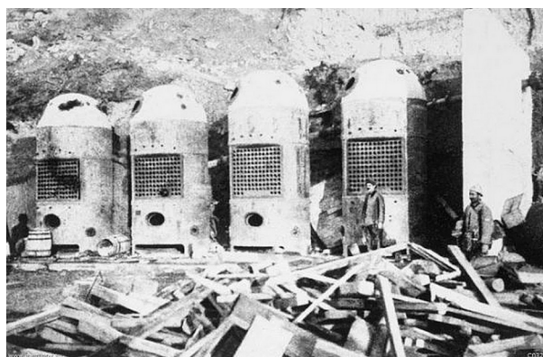
Fig. 5. Water purification system at AriBurnu
