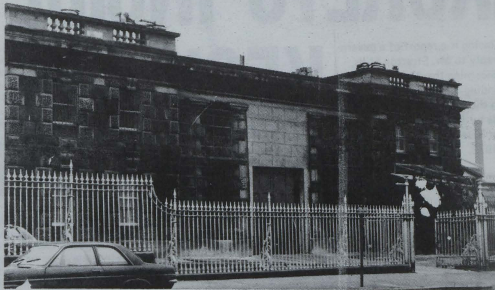
CRUMLIN ROAD PRISON, BELFAST
