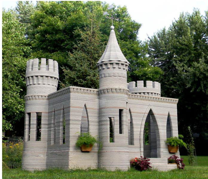
Figure 2.1 First 3D Printed Permanent Concrete Structure
