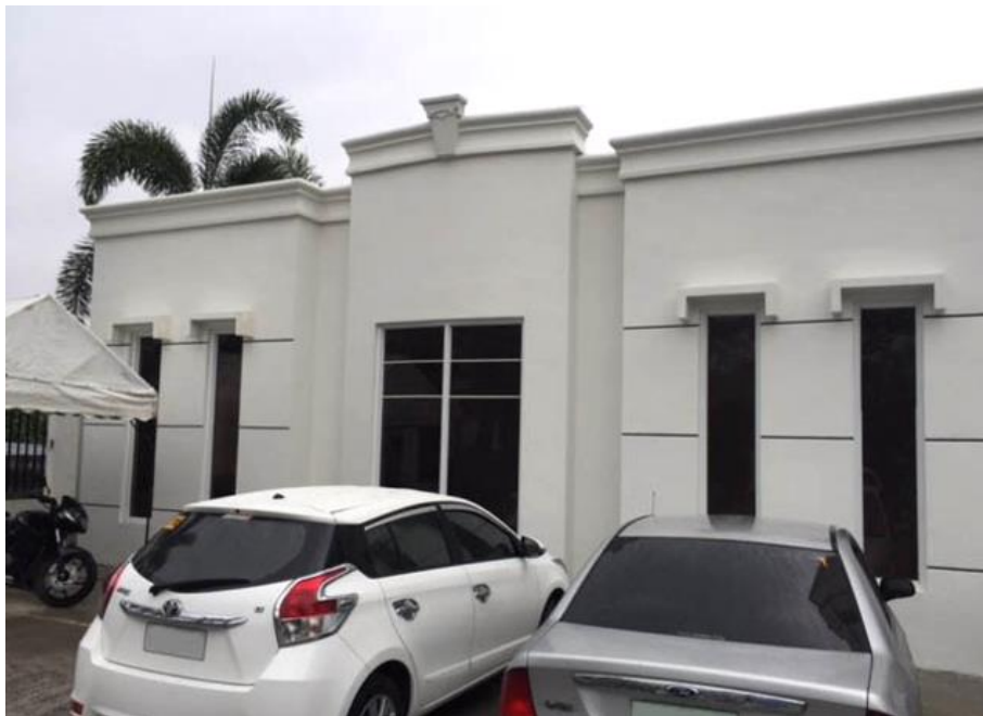
Figure 2.2 First 3D Printed Hotel Suite, Exterior
