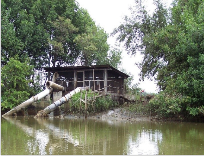
Figure 8. A Typical Ecuadorian Shrimp Pond Water Intake System. The pipes and pump located in the pump-house move water from the estuary to the shrimp pond. The shrimp pond is located behind the wooden pump house pictured. Picture taken near the village of Salinas on the northern side of Chone Estuary, January 2008.
