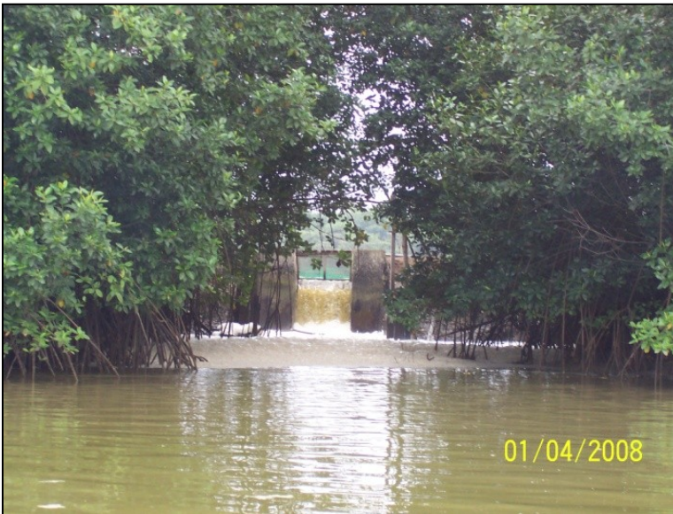
Figure 9. A Typical Ecuadorian Shrimp Pond Discharge System. The concrete and wooden damn returns water from the shrimp pond to the estuary. The shrimp pond is located behind the outflow pictured. Picture taken near the village of Salinas on the northern side of Chone Estuary, January 2008.
