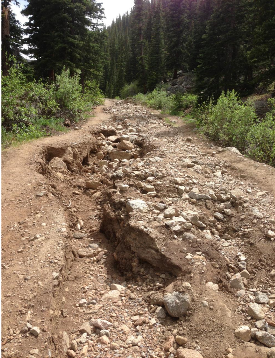
Figure 42. Mountain road washed out by recent storm. Under “normal” conditions, this road is passable in a 2WD car. Under the circumstances, this stretch may be impassable with a 4WD vehicle.
