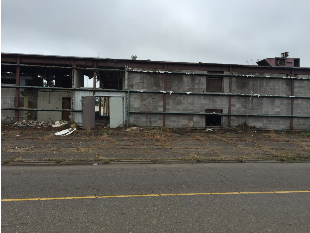
Figure 15. Dews Foundry Facing Edwards Street (Photo by author).
