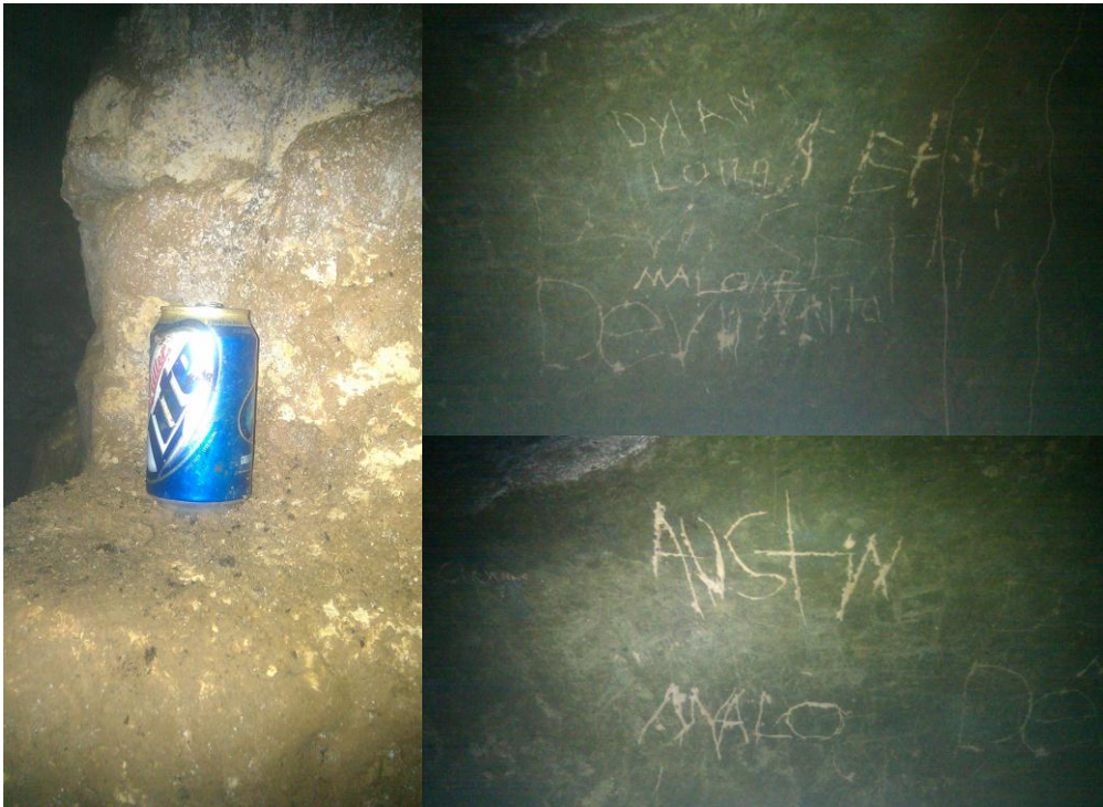
Figure 5. Vandalism in Pitts Cave. This picture shows trash and graffiti that are common to the entrance and tunnels of Mississippi's largest cave, Pitts Cave. The beer can in the picture is sitting exactly as it was found: upright on a limestone outcropping.
