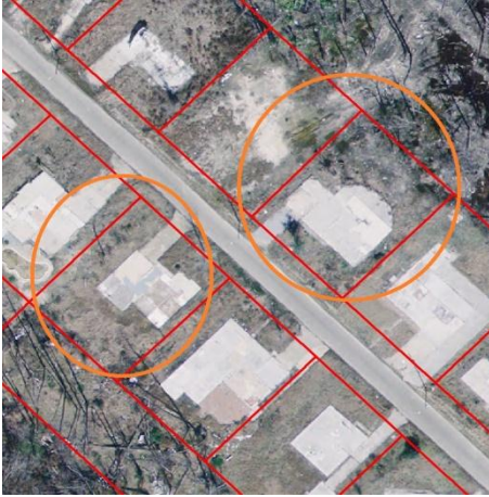
Figure 11: Empty slab (ES) shown highlighted in the orange area of interest. These parcels were identified by bare concrete slabs, where structures once stood.
