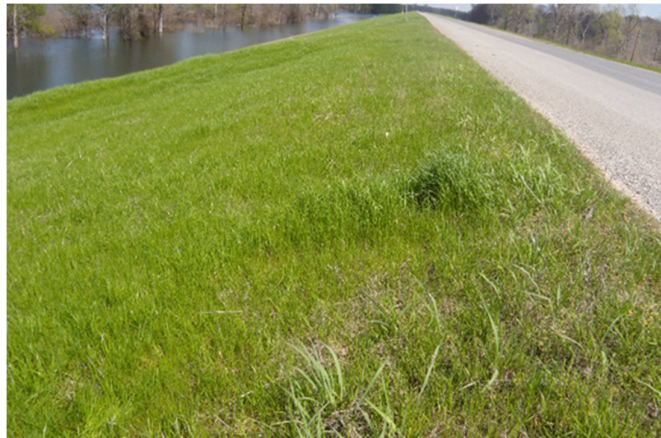
Figure 1. Earthen levee at Eagle Lake, Warren County, Vicksburg, MS, USA.
