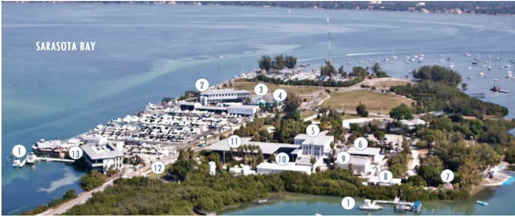
Fig. 14. Aerial view of the Laboratory’s main campus, Ken Thompson Park, City Island, 2010. 1. Boat Docks. 2. Goldstein Marine Mammal Center. 3. Dolphin, Whale and Sea Turtle Hospital. 4. Aquarium (marine mammals). 5. Main Research Laboratory. 6. Martin-Selby Immersion Theater. 7. Chickee. 8. Fish Stock Enhancement Experimental Center. 9. Elasmobranch Experimental Center. 10. Stein Fisheries Center. 11. Aquarium. 12. Martin-Selby Education Resource Center. 13. Keating Marine Education Center.
