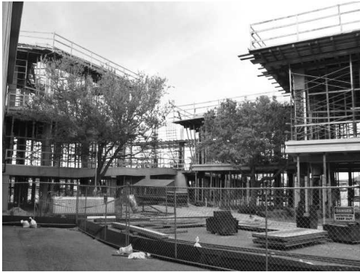
Fig. 18. Expansion of the Institute in 2011. The Estuarine Research Center under construction.
