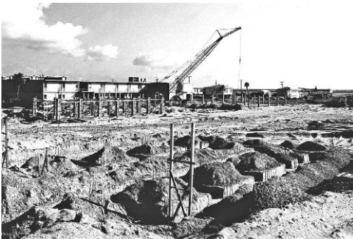
Fig. 3. Expansion of the Institute in the 1970s.
