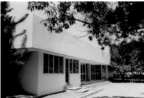
Fig. 2. Main entrance to the administrative building.
