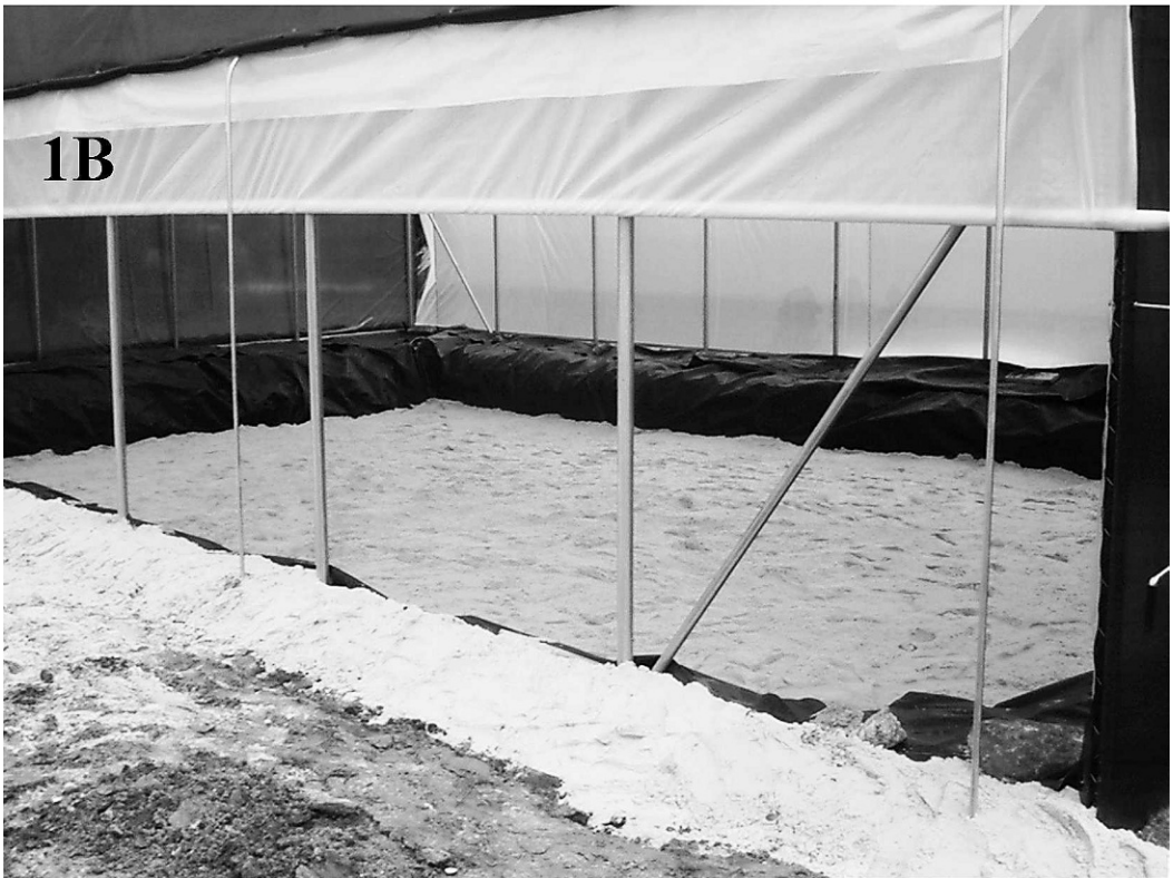
Fig. 1. Photographs of the land-based seagrass nursery at the Cockroach Bay Aquatic Preserve in Ruskin, FL. (A) Pole building with the fiberglass side screens rolled down. (B) View from outside the building with a side screen rolled up, showing the 10–20-cm layer of coarse sand covering the Permalon™ vinyl liner in the 74.4-m 2 basin.
