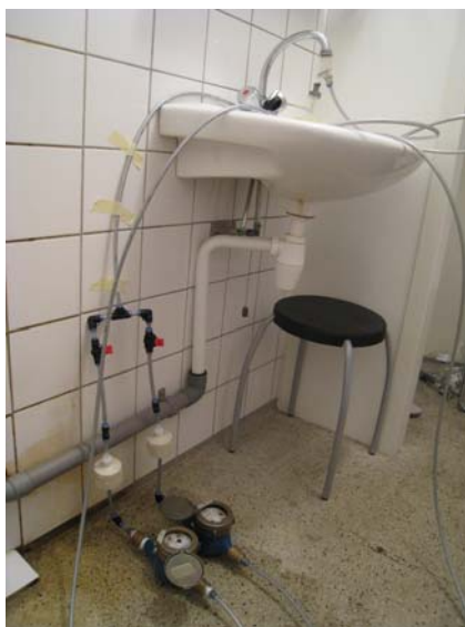
Figure 6.19. Installation of the MuPFiS at the consumer's house in Delft.
