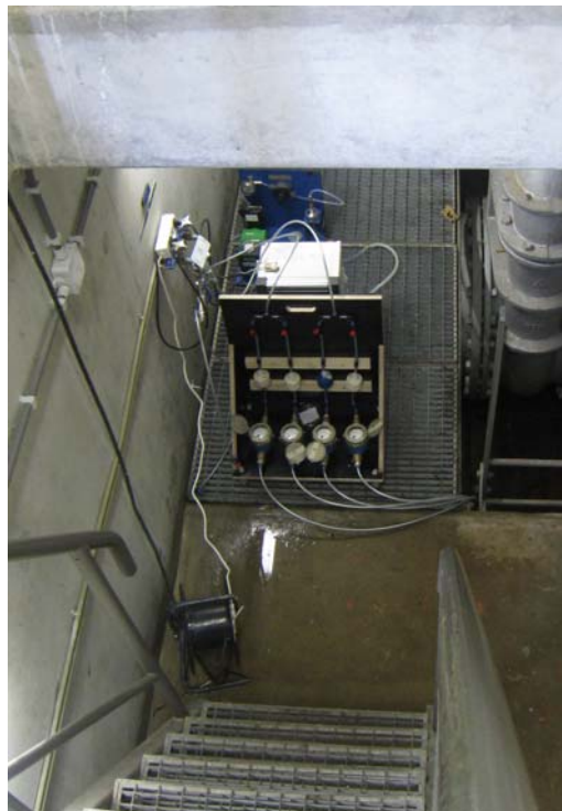
Figure 6.9. Installation of the MuPFiS and TILVS at the Amstelveenseweg North line.
