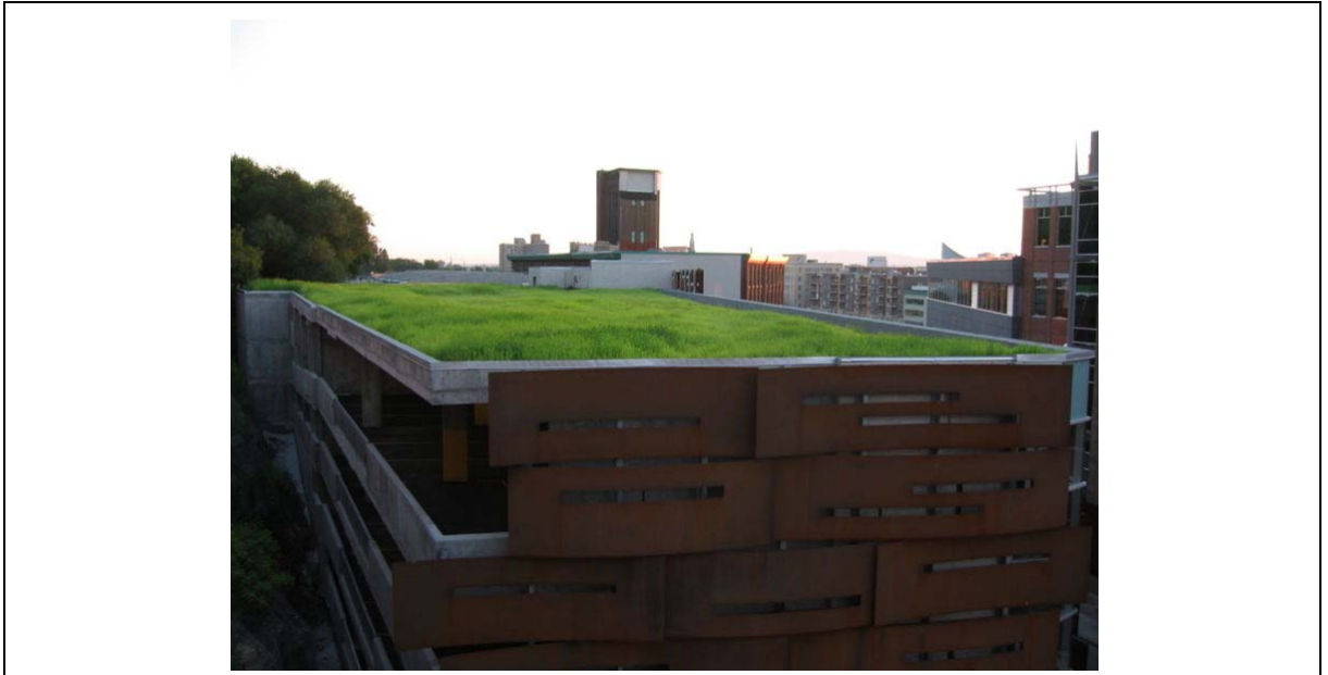
Figure 46: Flat green roof
