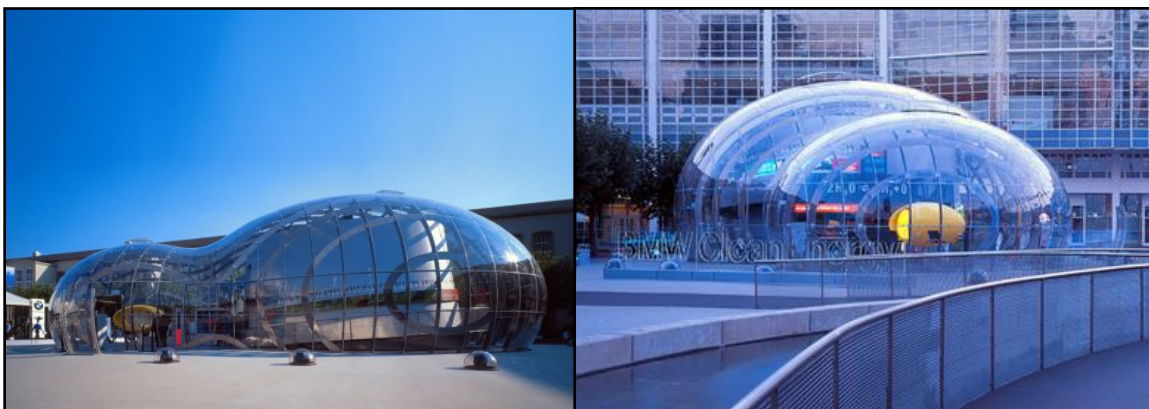
Figure 0.1: Pavilion designed for the presentation of the BMW group at the International Automobile show IAA 1999. Its double curved shell made of crystal clear acrylic glass was manufactured thanks to a computer-controlled process.
