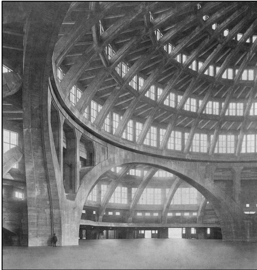
Figure 1.8: Interior view of the Breslauer Jahrhunderthalle, built in 1913. This 65 m spread steel-concrete dome with a ribbed structure represents a transition between the massive domes and the new shell domes that would appear in the following years. It was designed by the Dyckerhoff & Widmann AG office.
