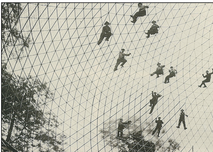
Figure 1.7: The innovative idea of a new conception system: the steel mesh of the 25 m diameter planetarium in Jena. This kind of structure can support great charges suffering a minimal deformation, as we will see in the following chapter.
