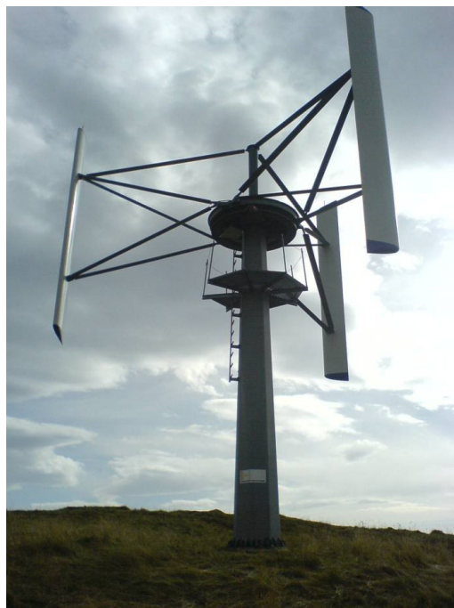
Figure 4.1.4. H-rotor Darrieus Giromill wind turbine with 10 m diameter in RotwanHaus (Bayern Germany).
