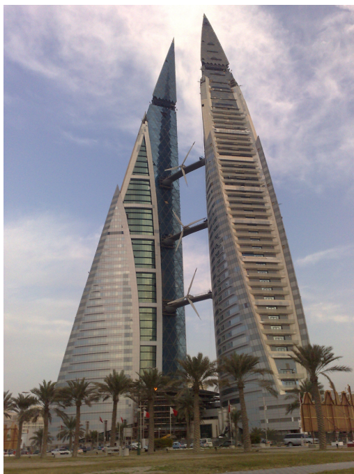
Figure 4.2.5. Three 225 kW, 3 bladed HAWT mounted between the towers of the Bahrain World Trade Centre. 2008.
