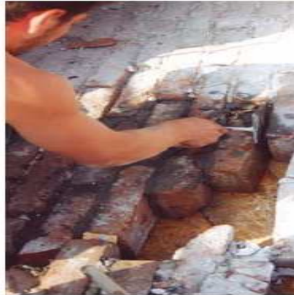
a. Preparation of the surfaces
