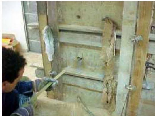
Figure 3.22: Strengthening of Columns (Tumialan et al. 2001).
