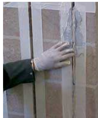
(b) Encapsulation of FRP Bar
