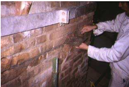
(c) Refilling by the repointing material
