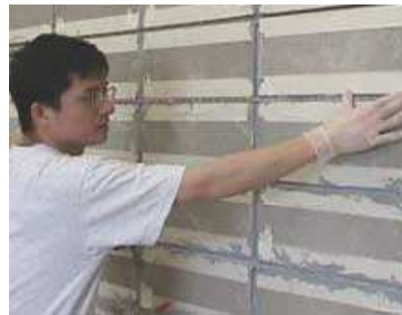
(b) Installation of GFRP Bars
