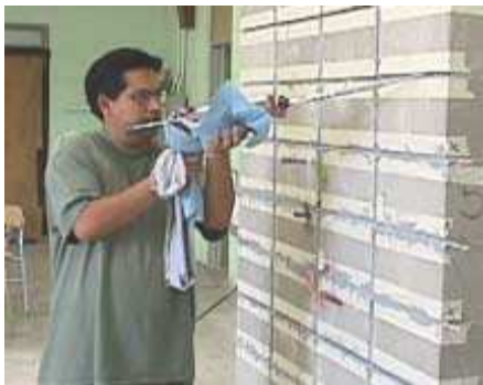
a) Application of Embedding Paste
