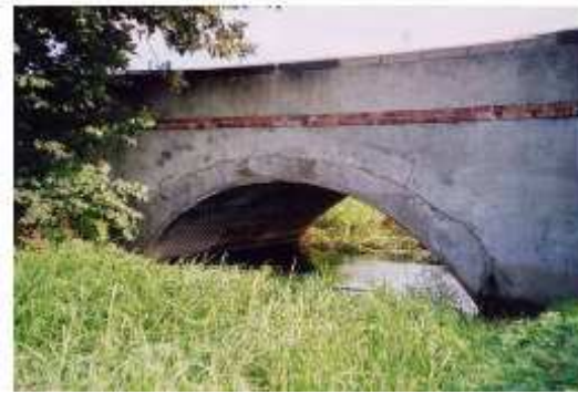
Figure 2.5: Bridge strengthened with external steel strips (Lorenzo Jurina)
