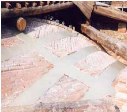
c. After Application of FRP
