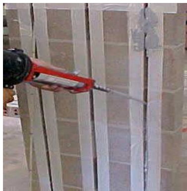
(a) Application of Embedding Paste
