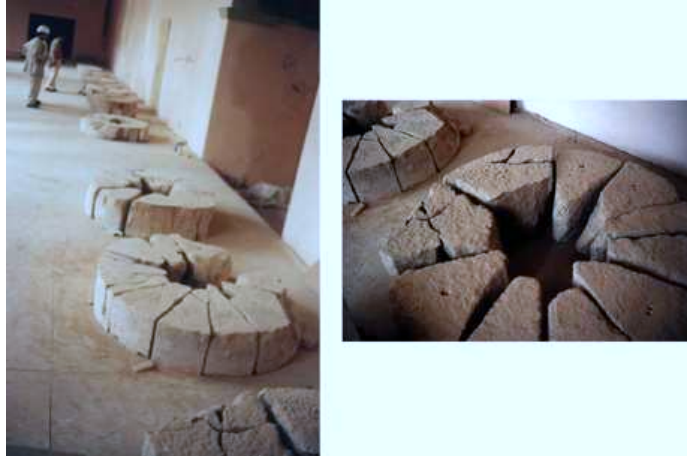
Figure 2.10: Removal of a pier of Tarazona Cathedral, Spain. (EU-India cross program, 2006)
