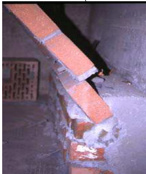
Figure 3.28: Failure mechanism detected in tests (sliding failure) (Valluzzi et al. 2001)
