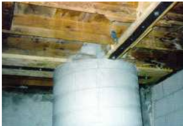
Figure 2.28: Parallel System of Foundation Repair (California seismic society, 2005)
