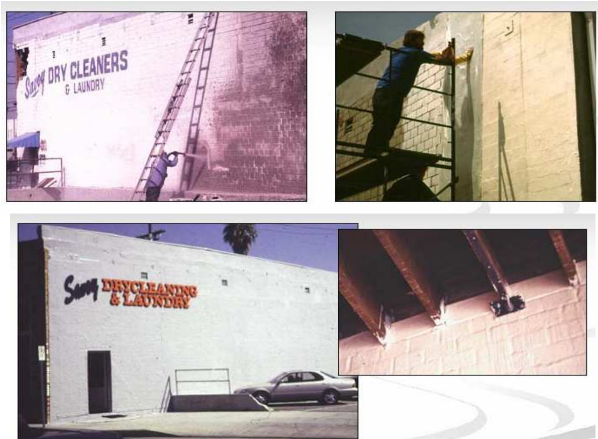
Figure 3.15: One-Story CMU Block Building, Glendale, CA (QuakeWrap, Inc.)
