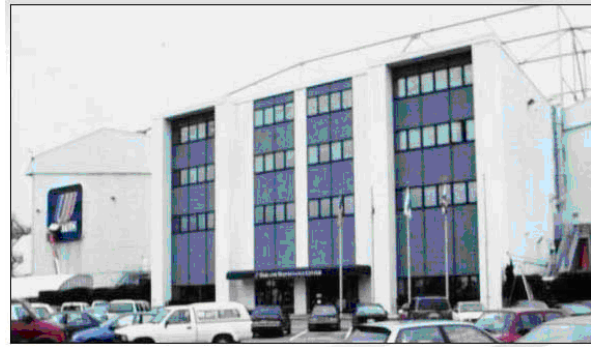
Figure 3.17: United Airlines Building, Oakland International Airport. (QuakeWrap, Inc.)
