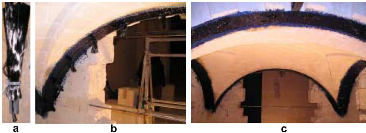
Figure 3.31: Strengthening of the vaults with FRP sheet. (a) FRP spike; (b) the spikes are inserted through the sheet into the holes; (c) picture of the vault after completion of strengthening. (Lorenzis et al, 2007)
