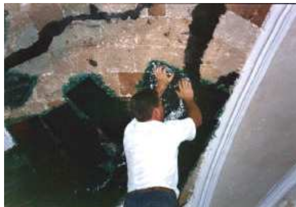
Figure 3.38: Strengthening of Masonry Vaults (Tumialan et al, 2001).
