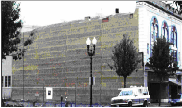
Figure 3.16: Two-Story Masonry Building, Redwood City, CA (QuakeWrap, Inc.)
