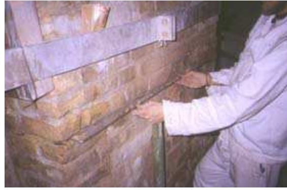
(b) insertion of reinforcing bars in the bed
