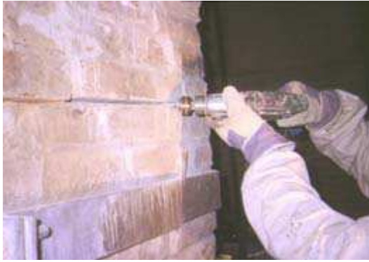
(a) excavation of the mortar joint
