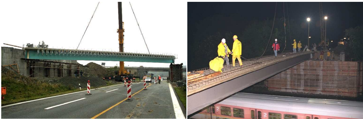
Fig. 4.1. VFT girders assembly over active road and railway track.
