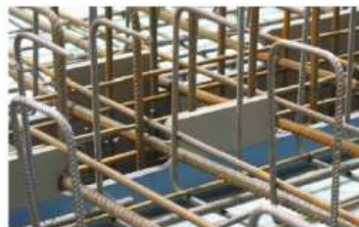
Fig. 13.7. Reinforcement for prefabricated concrete plate
