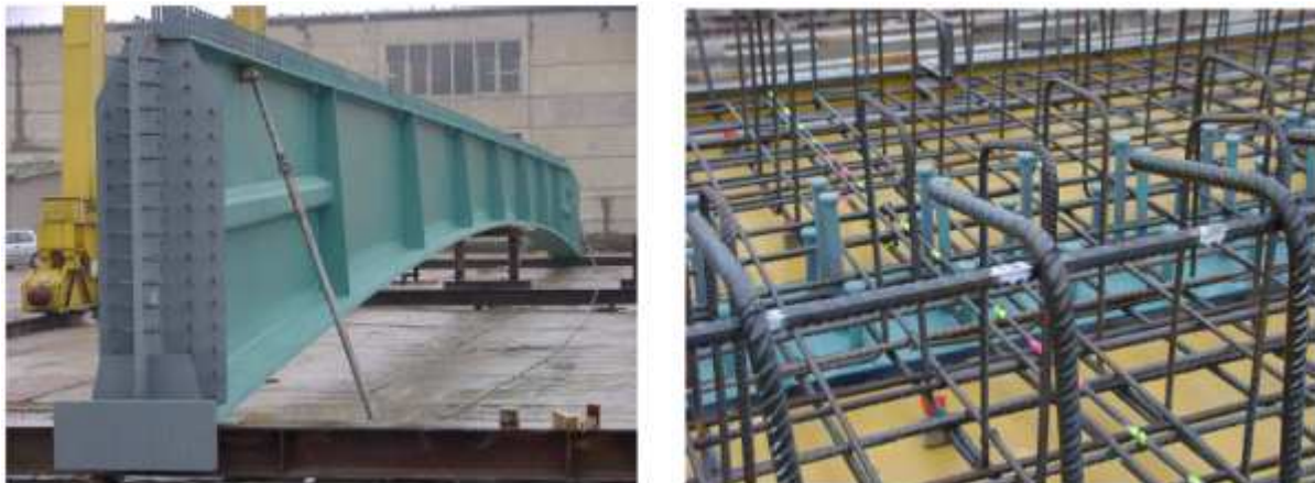
Fig. 5.2. Steel girder in factory, stud shear connectors and prefabricated slab reinforcement .
