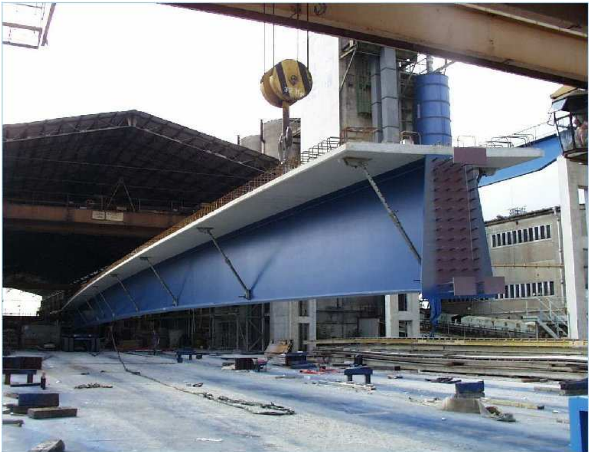
Fig. 5.4. "Ready to transportation" VFT girder in the factory.
