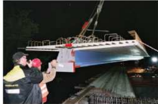
Fig. 13.9. Placing of the VFT-WIB girder with 32,50m length
