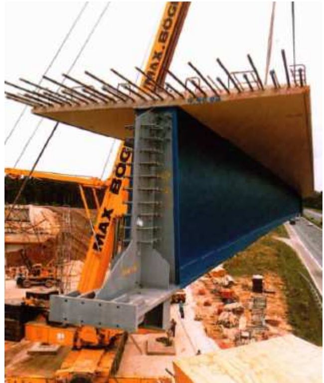
Fig. 6.1. Girder assembly by crane.
