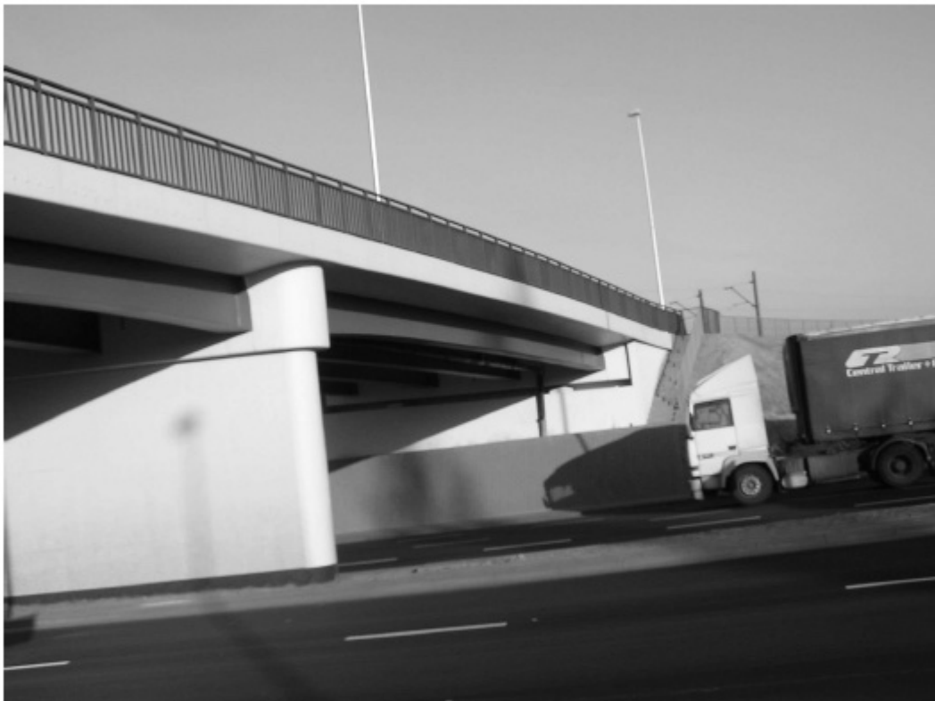
Figure 9.1. Bridge view (Szczecin – Struga Avenue).
