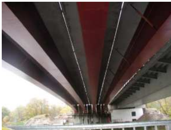
Fig. 3.9. Cross section with 4 VFT girders.
