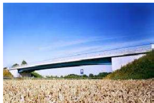
Fig. 4.2. Frame viaduct VFT over the motorway.
