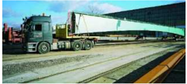
Figure 5.3. VFT girder transportation
