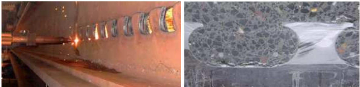
Fig.13.3. Cutting line of the web.
