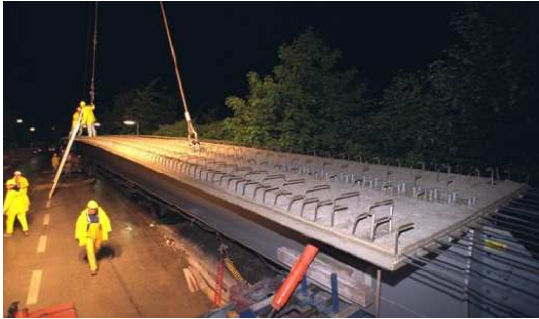
Fig. 6.4. VFT unit assembly during the night.
