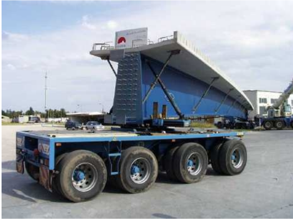
Fig. 6.2. Transport of VFT girder.
