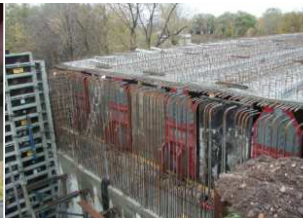
Fig. 3.10. Beams support the abutment directly.
