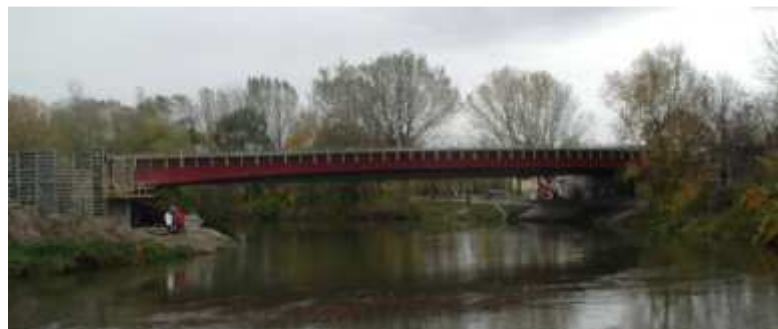
Fig. 3.11. View of bridge across the river Saale in Merseburg.
