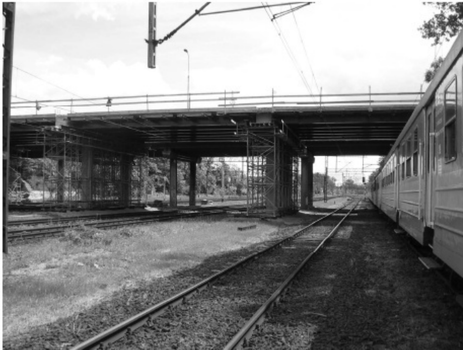
Fig. 9.5. Bridge view during construction phase (Wrocław-Armii Krajowej Avenue).
