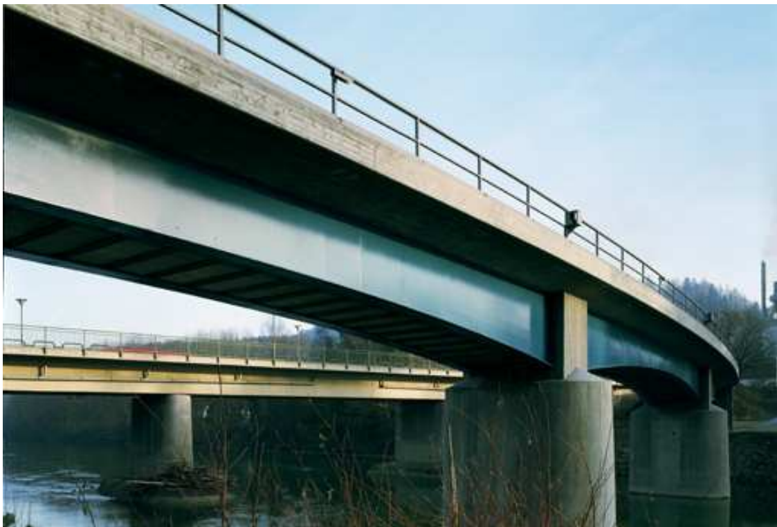
Fig. 3.12. View of the bridge across the river Lech in Schongau.
