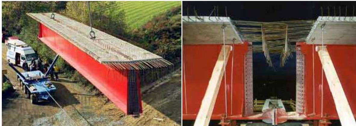
Figure 6.3. Lifting and laying of the VFT prefabricated units.
