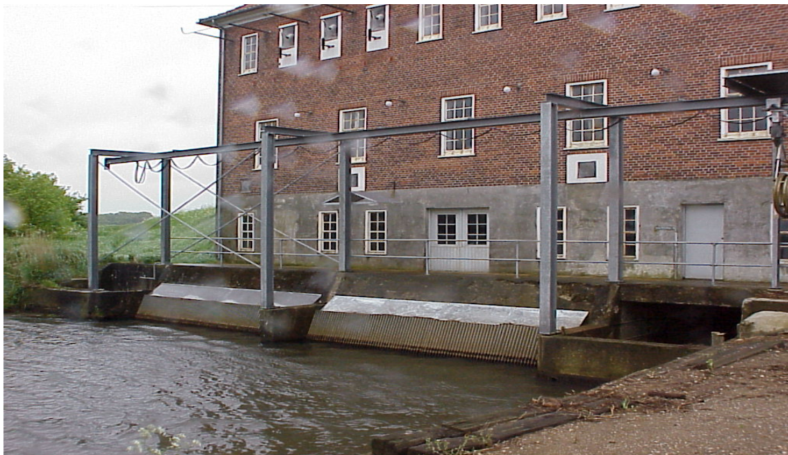
Figure 2 - Tønder's pump station
