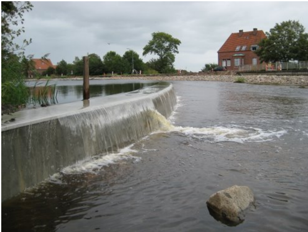
Figure 21 – Vidaa River Control Station
