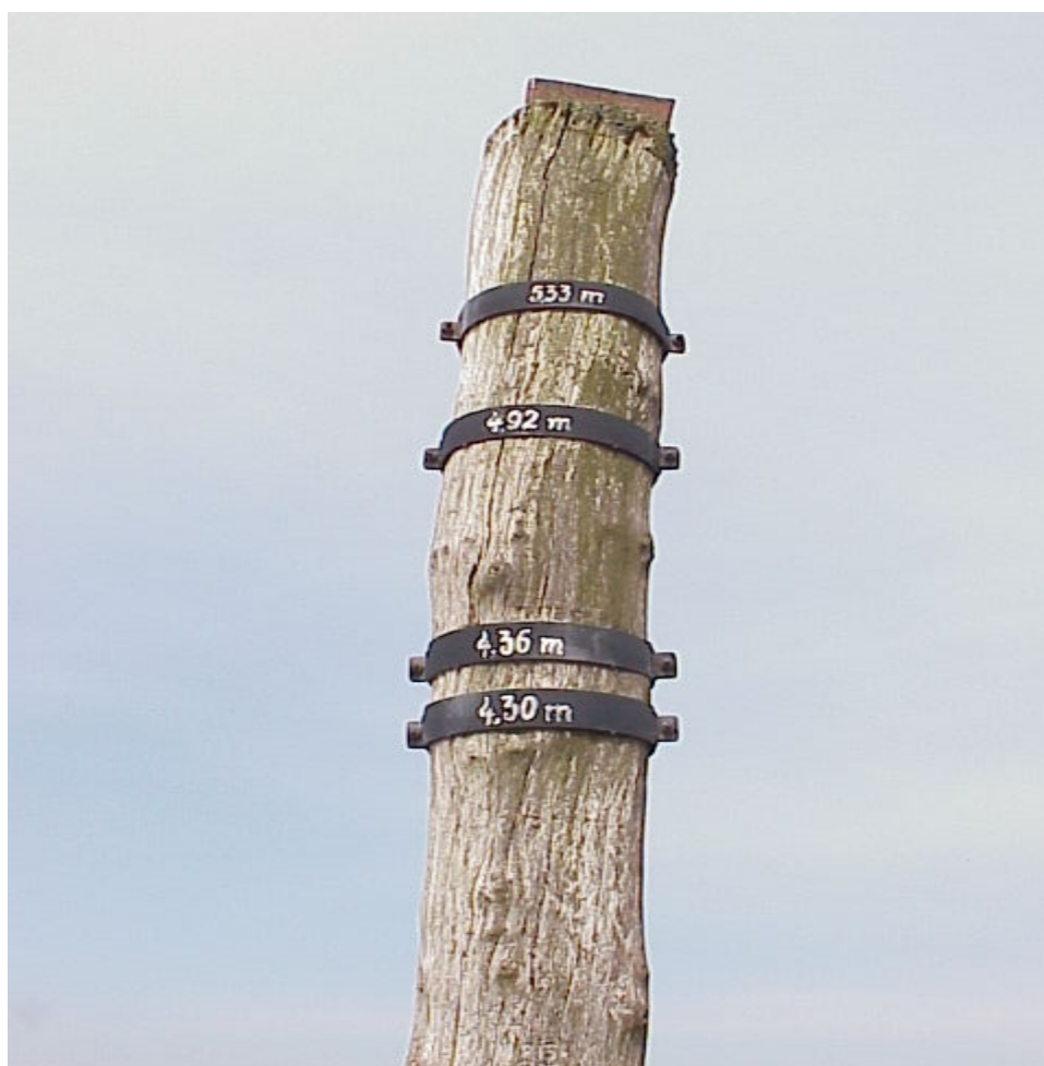
Figure 5 – Rings on a storm flood pillar at the sluice in front of the old Højerdiget dyke
