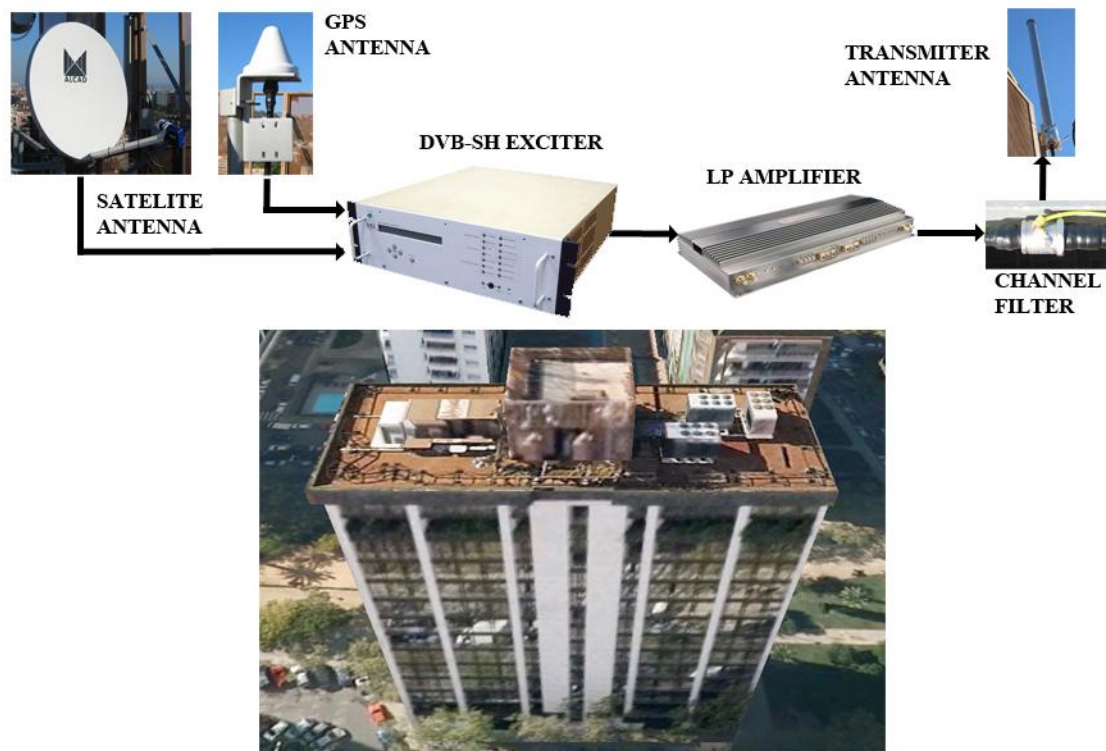
Figure 3.2 Equipment installed in Pere i pons site
