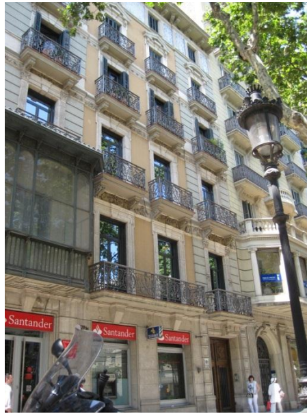
Figure 5.6: Façade of 629 Gran Via de la Catalanes
