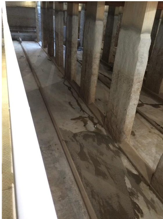
Figure 15. Inside of the tank. First visit.
