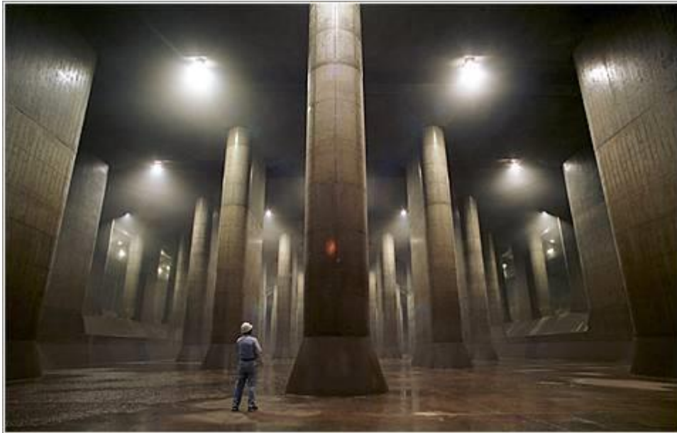
Figure 3. An example of a retention tank in the drainage networks in Tokyo.
