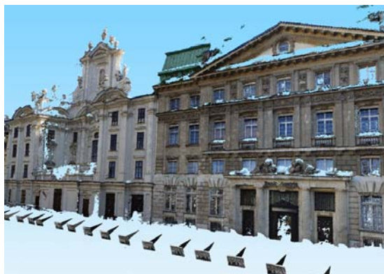
Figure 7: Dense textured point cloud calculated using the information from the oriented sequence of images shown in the front of the façade.
